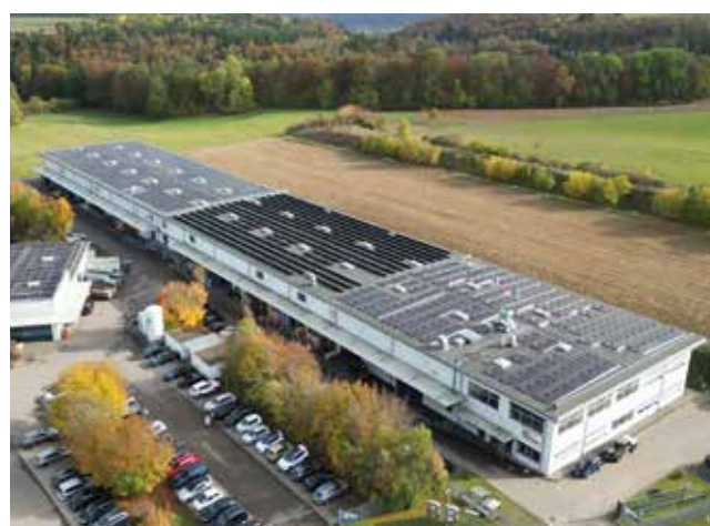
Picture above: 180 new storage spaces have already been created Picture below: Photovoltaic system with an output of 521 kWp
