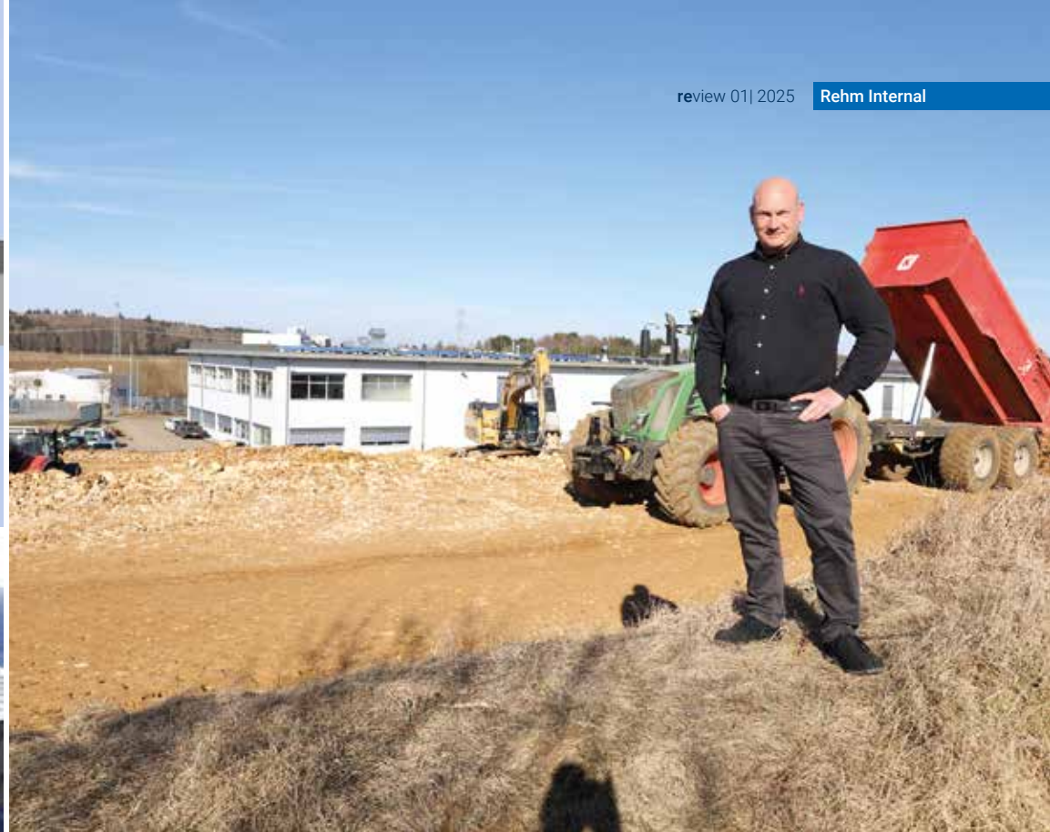
The first construction phase for the new extension of Rehm BlechTec is almost complete.
