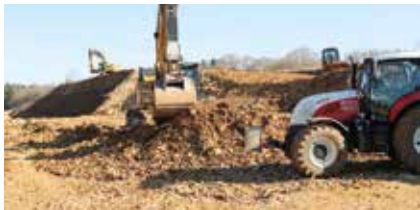
Construction work for the extension of Rehm BlechTec has begun
